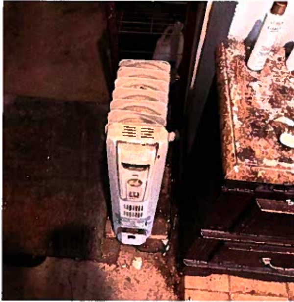
(Photograph of electric space heater in bathroom. Taken by Detective John Agnew.)
