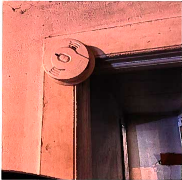
(Photograph of only working smoke detector on property. Taken by Detective John Agnew.)
